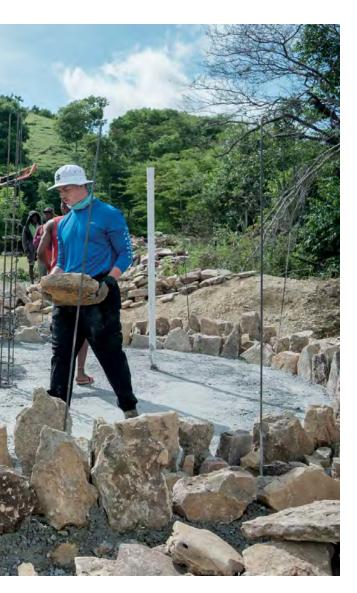
Clockwise from lower left, the Mercer group and local residents examine the existing spring box and piping for damage and assess the water level prior to building a new water system; the Mercer group and local residents carry stones for a new water tank; the Mercer group and local residents use stones to build the tank.
