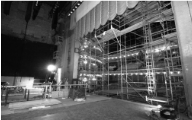
ABOVE: The Grand Opera House underwent a complete repainting during renovations that included a new color scheme. BELOW RIGHT: The renovation project called for the replacement of the original stage floor. Scaffolding was constructed inside the theater for the repainting job to be accomplished.
